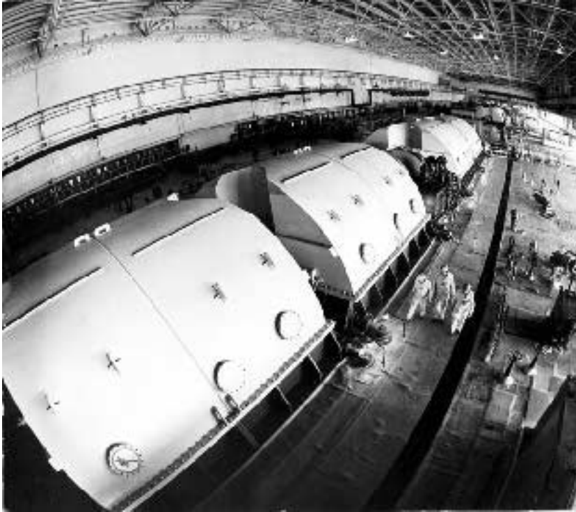
Figure 2.3. Turbine hall, November 1982. (Courtesy: TASS.)
